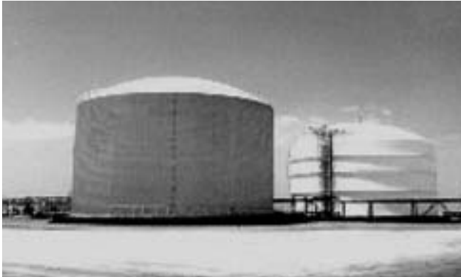
A flat-bottomed cylindrical single shell tank for storing liquefied butane gas is one recent application for NB-1SJ, when constructed per BS7777 specification requiring -50^{\circ}\text{C} notch toughness based on fracture mechanics (Photo courtesy of Toyo Kanetsu K.K., Japan).
