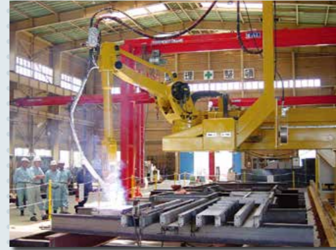
Bridge and Water Gates – ⑤
