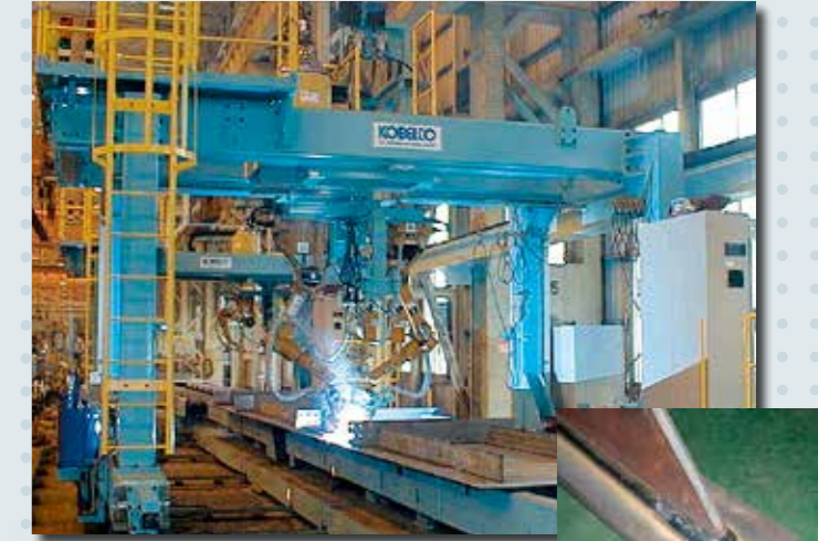
Twin Gantry Type System for Bridge Panel – ⑥
