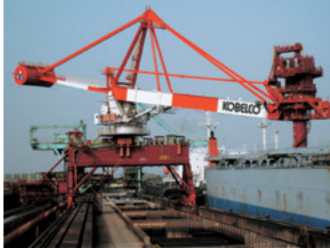
Ore & Coal Wharf
