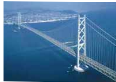
Akashi Kaikyo Bridge and ultra-high strength main rope
