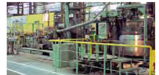
SV (SHAVELITE wire rod surface peeling) line
