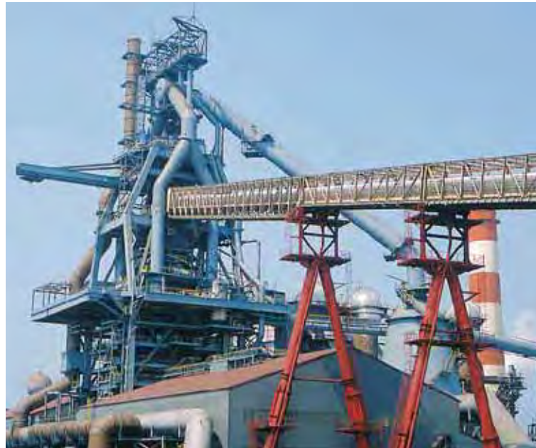
No. 3 Blast furnace
