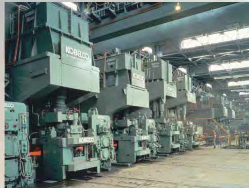
Roughing train Hot steel is passed through the grooved rolls to reduce its cross-sectional area.
