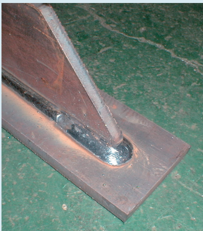
角巻溶接例(スニップ) Boxing Weld Bead Appearance (Snip Weld)
