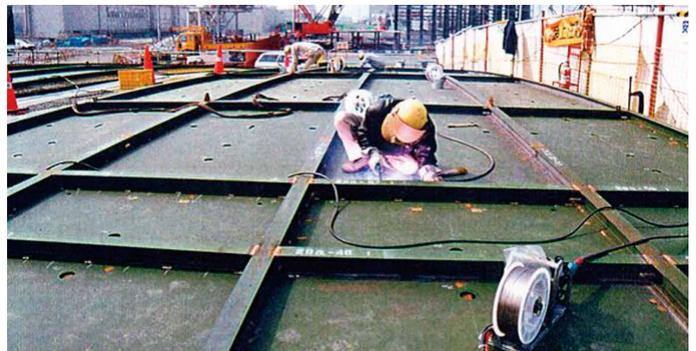
FCAW with DW-N70S / Horizontal Fillet Welding at Roof Plate
