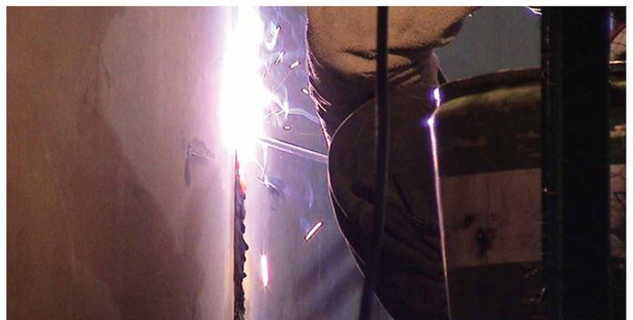
SMAW with NI-C70S / Vertical Upward Welding at Side Plate
