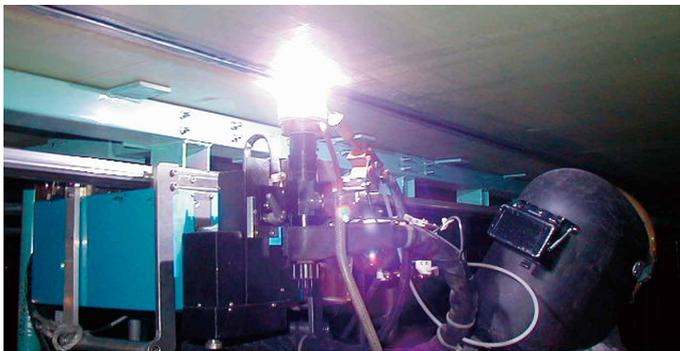
AUTO- GTAW with TG-S709S / Overhead Welding at Bottom Plate
